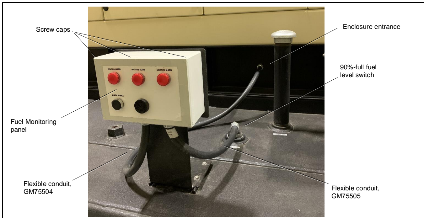
Figure 50 Fuel Monitoring Panel, Overview
